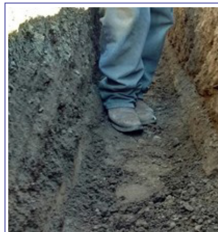
Figure 5. Three-foot trench with a gopher tunnel system at the base illustrates the lack of effectiveness of fencing for keeping gophers out of fields (photo by D. Hannaford.)
